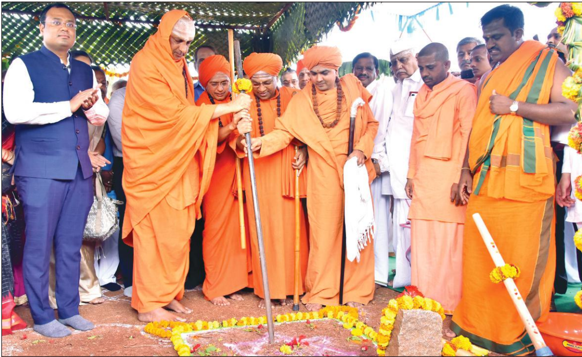
The foundation laying function of JSS Speech & Hearing College and Hostel buildings at Kelageri, Dharwad was held in gracious presence of HH Jagadguruji. Sri Nitish Patil, Deputy Commissioner, Jagadguruji of Sri Murusavira Math, Hubli, Jagadguruji of Sri Tontadarya Math, Gadag, Jagadguruji of Sri Shivananda Math, Sri G.S.Gaddedevaramath, Ex-MLA and others were present (5.4.2022)
